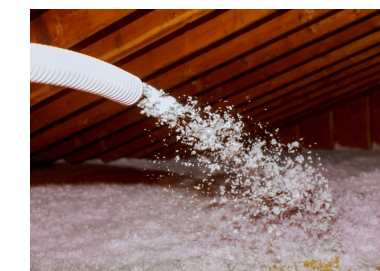
Insulation added to attic space
