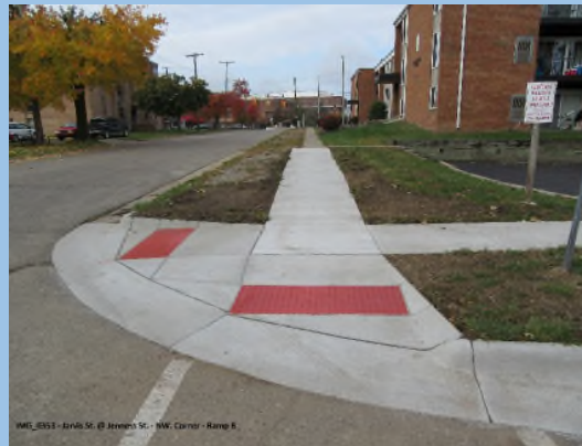
ADA Sidewalk ramps (City of Ypsilanti)
