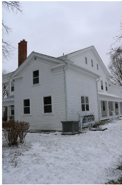
North wing, rear elevation
