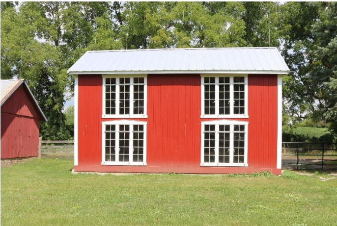
Rebuilt Pig Barn, front elevation, September 2020
