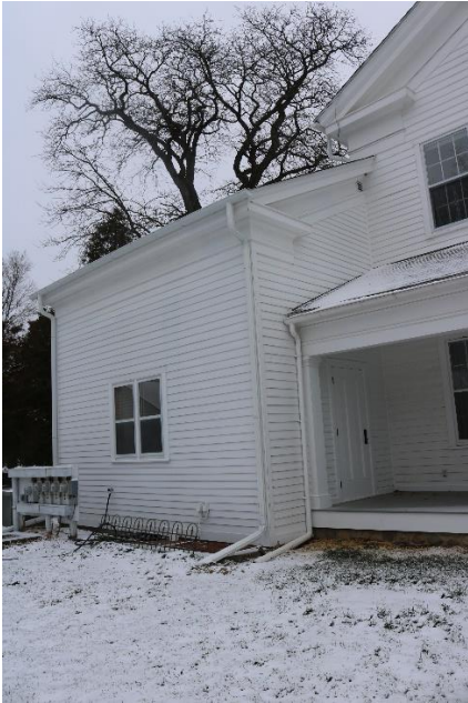
North wing, door on to rear porch door
