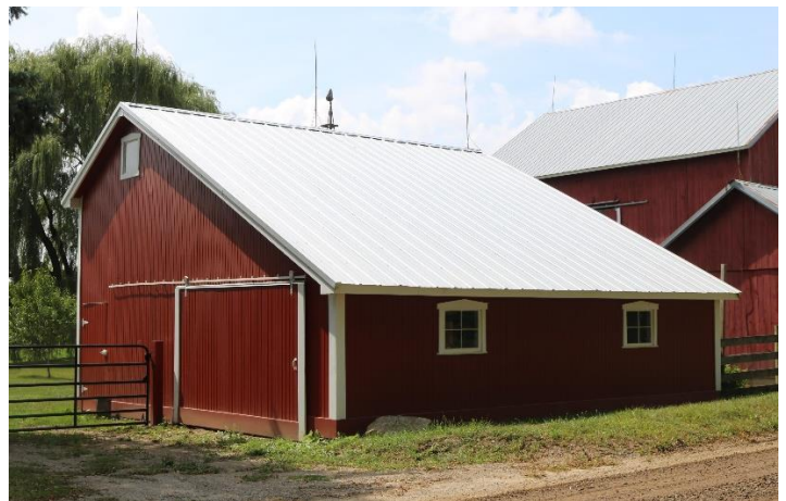
Rebuilt Pig Barn, rear, September 2020
