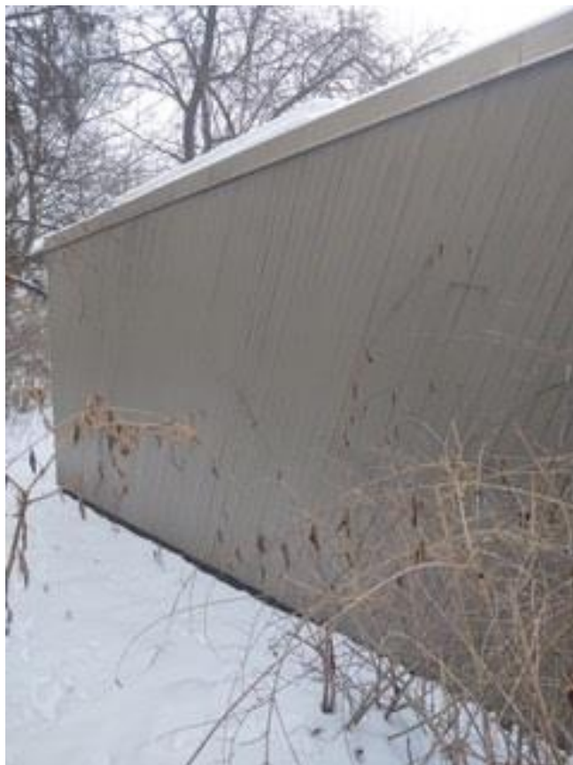
Garage side (south) elevation
