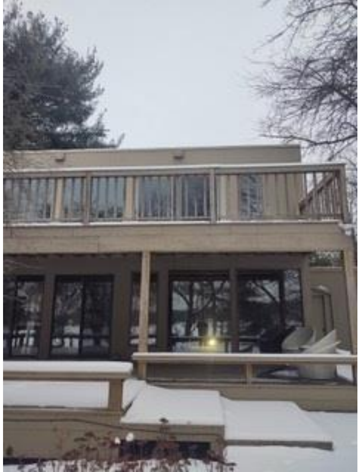
South end of rear (west) elevation
