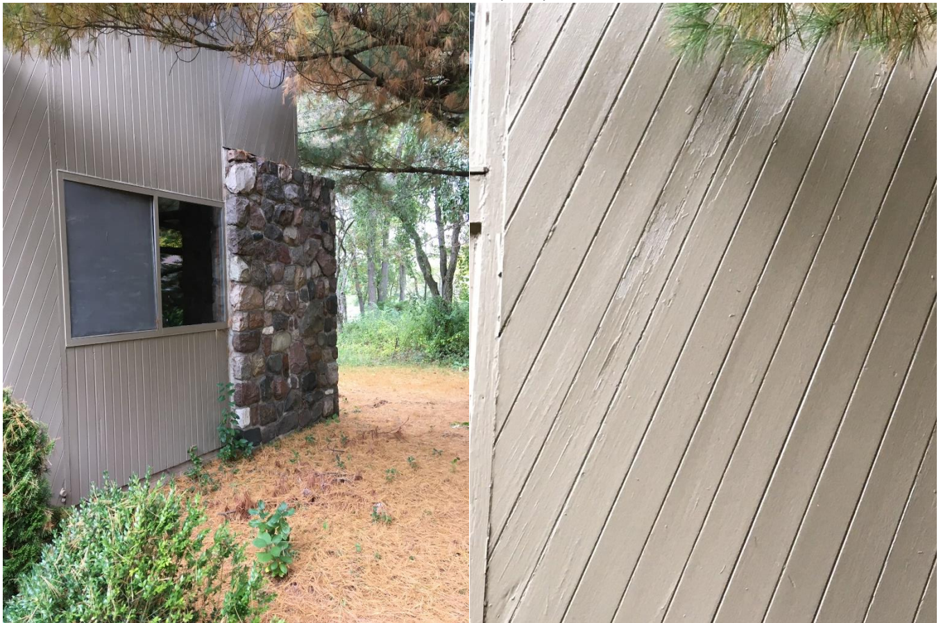
North end of front (east) facade, close ups
