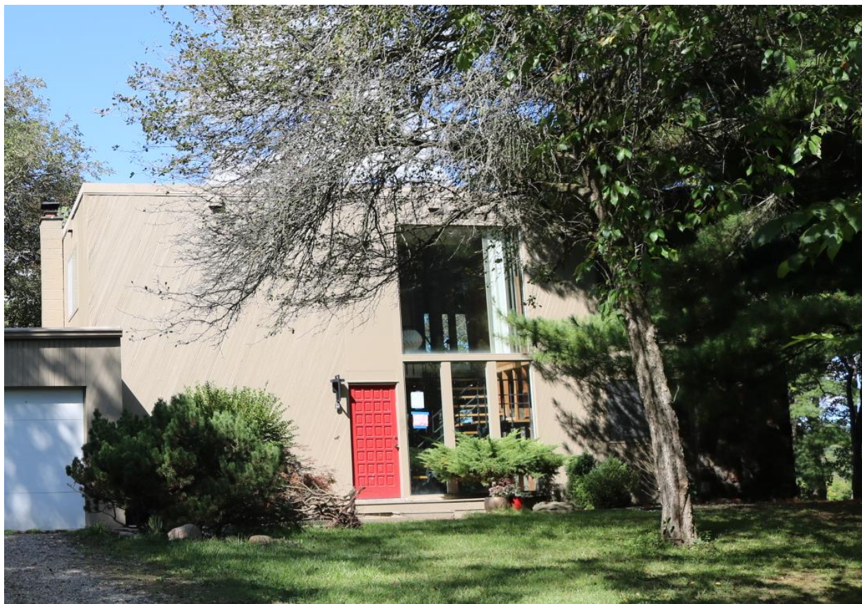
Front (east) facade, 4071 Thornoaks Drive
