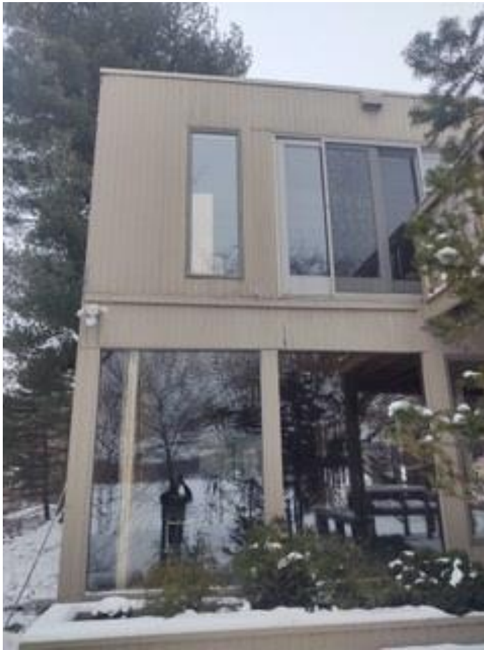
North end of rear (west) elevation
