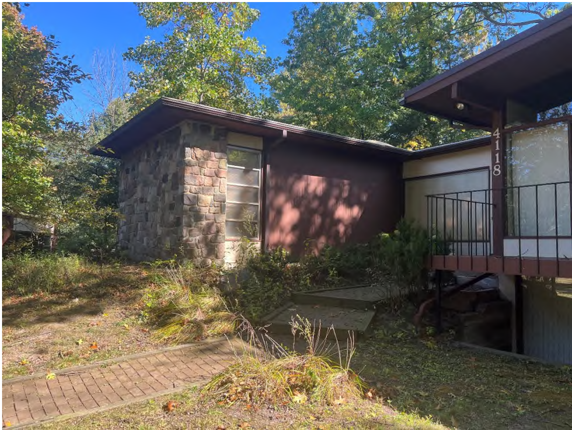
East half of front facade, view facing southeast. The rockface continues around onto a portion of the east elevation (see previous picture)
