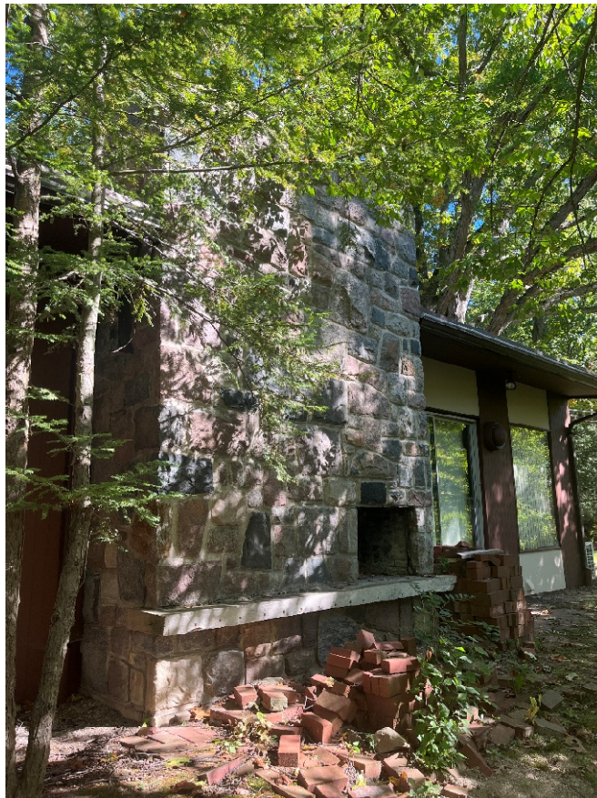
Chimney on west elevation
