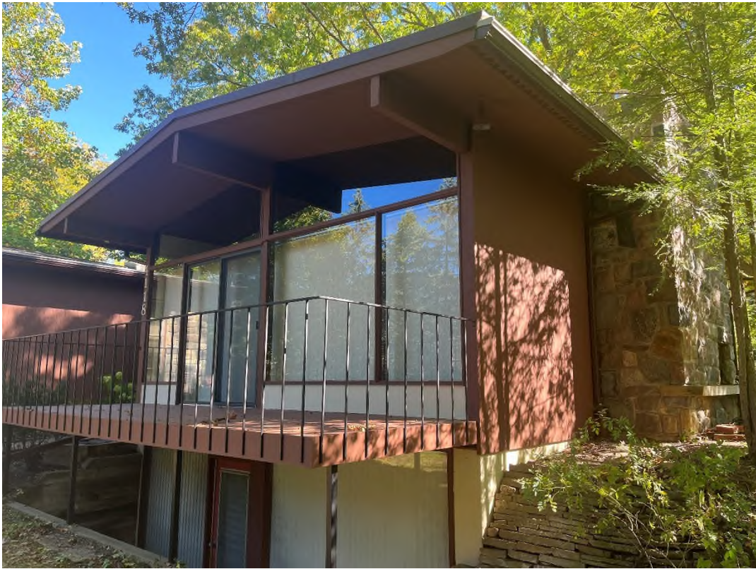
Front facade and west elevation, view facing southwest
