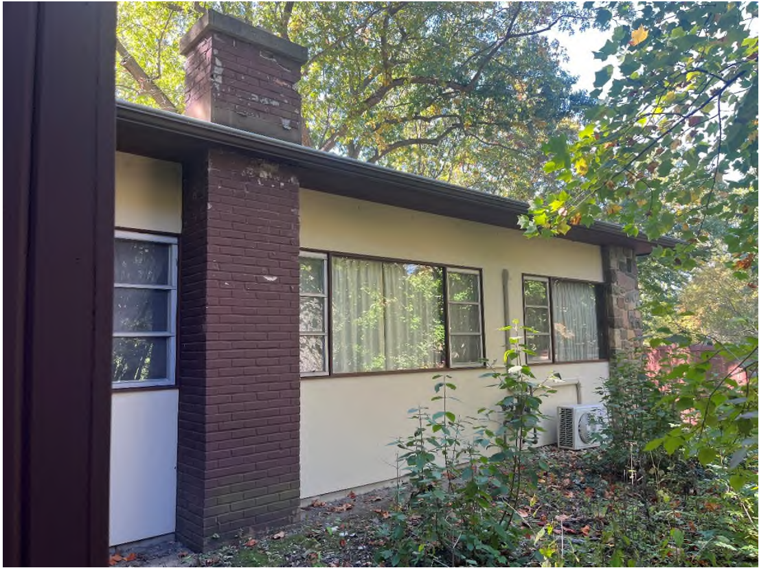
Project site, east elevation, view facing northwest
