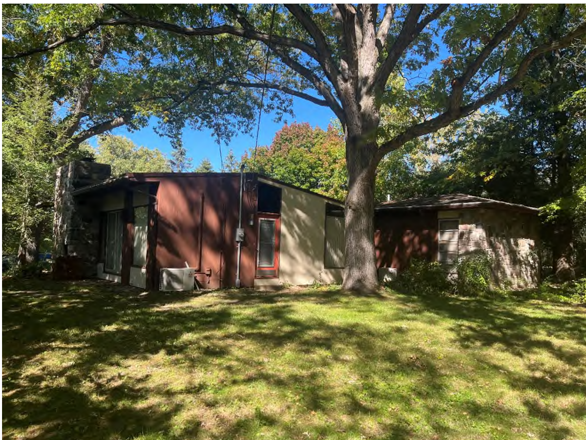
Rear (south) elevation, with view of west elevation and stone chimney, view facing northeast
