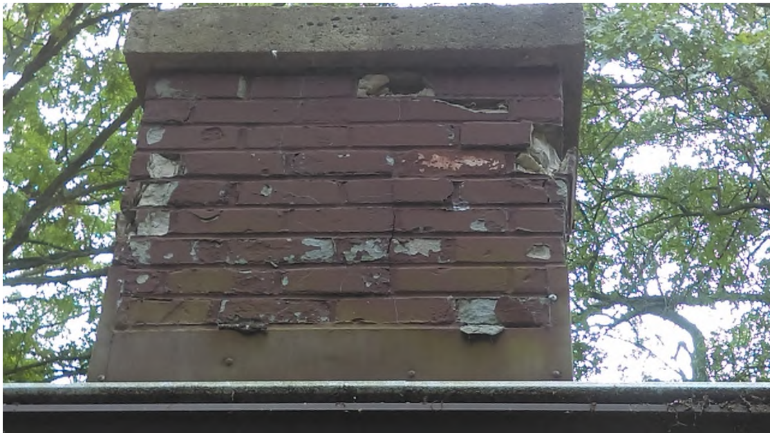
Portion of chimney proposed for removal
