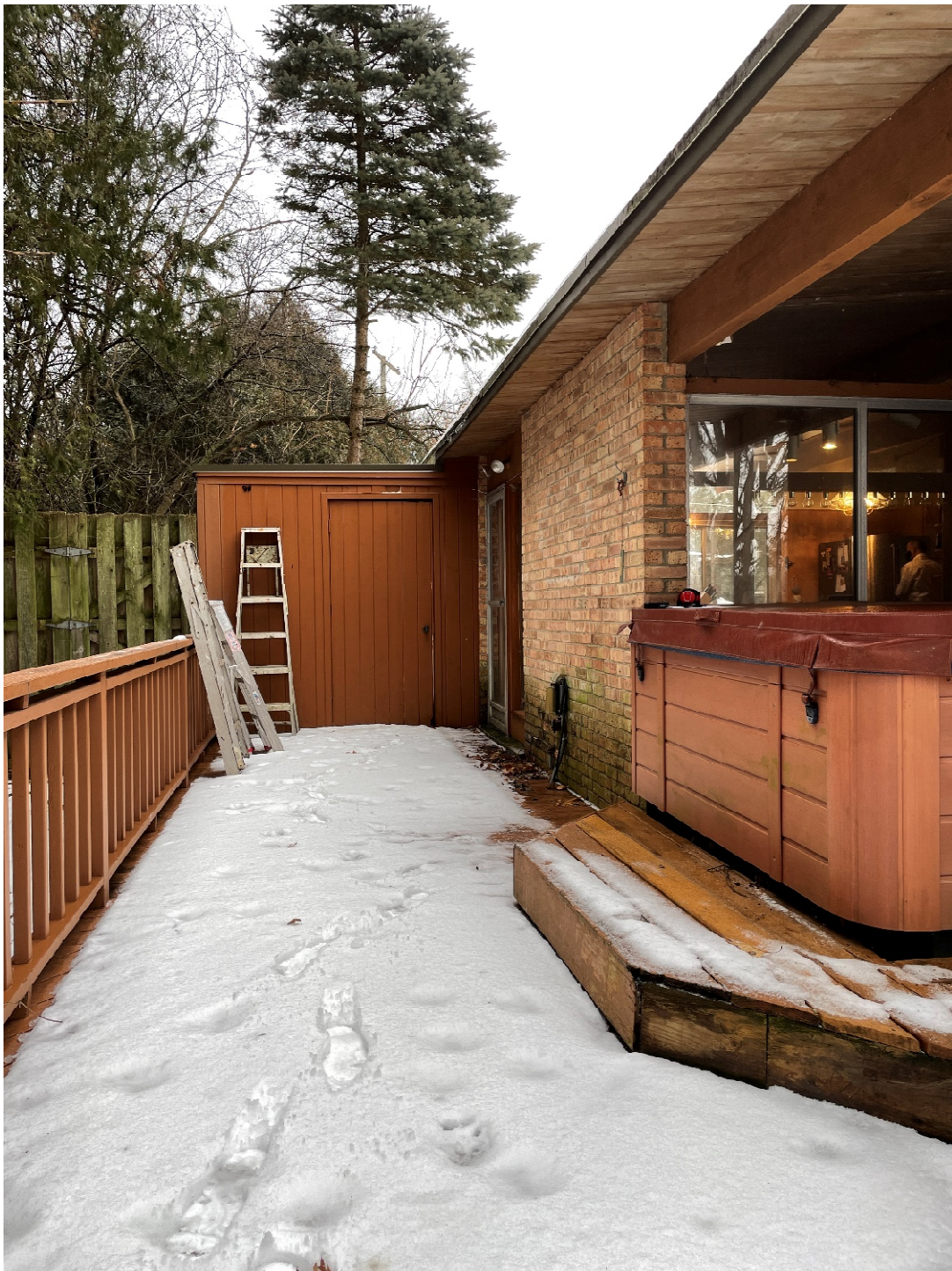
View of proposed location for the addition along north elevation, from the rear deck
