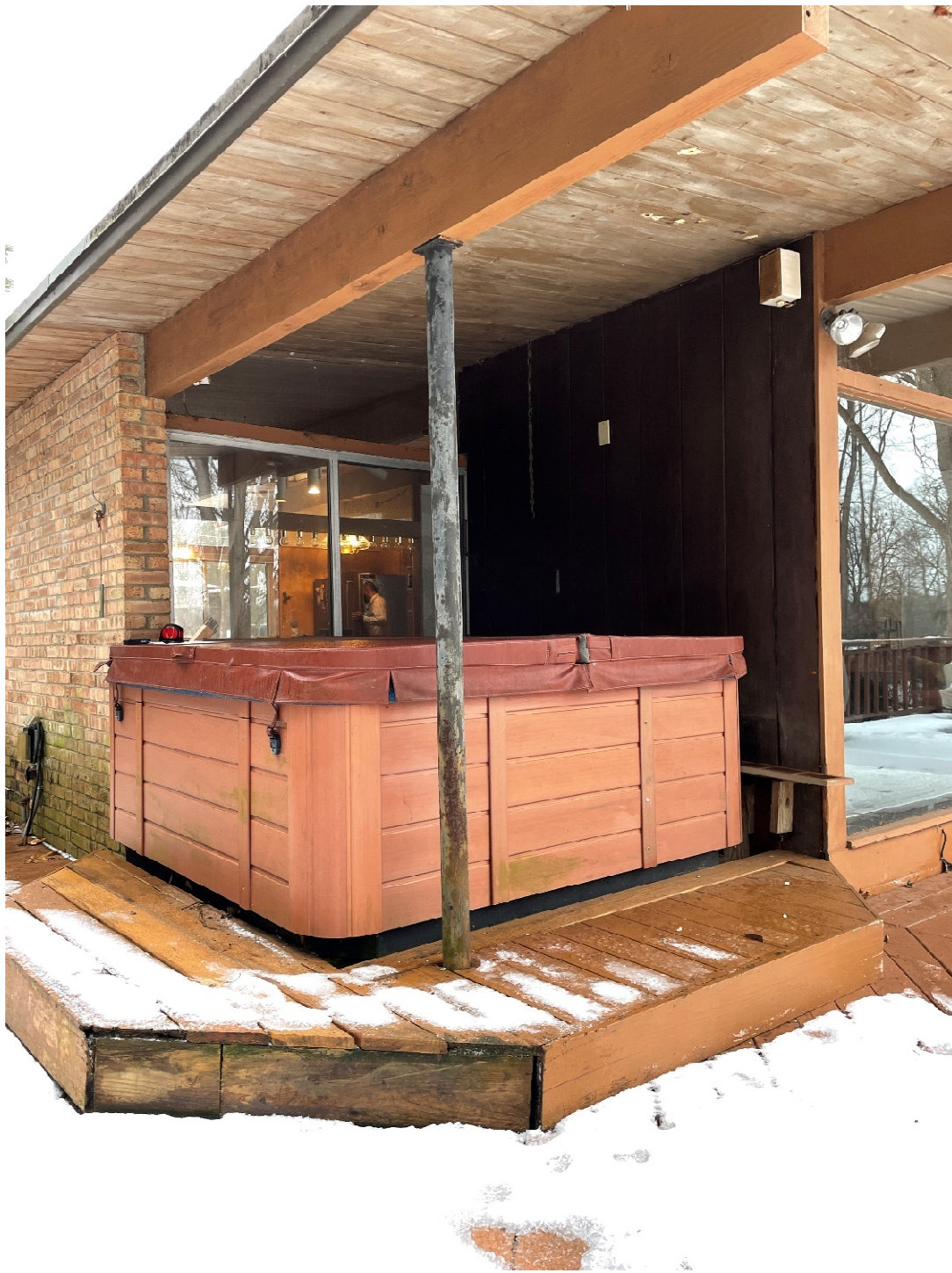
Rear elevation adjacent to the proposed location of the addition
