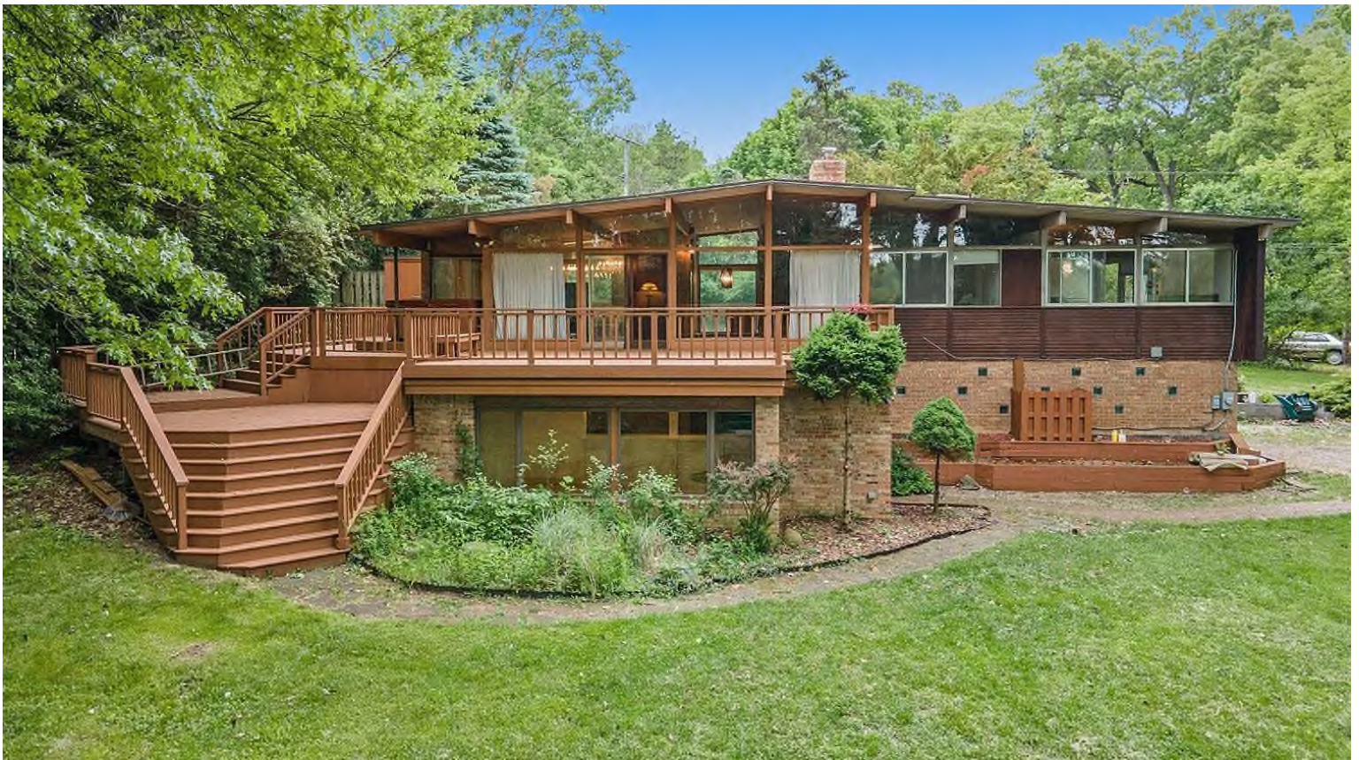
4101 Thornoaks Drive rear (west) elevation
