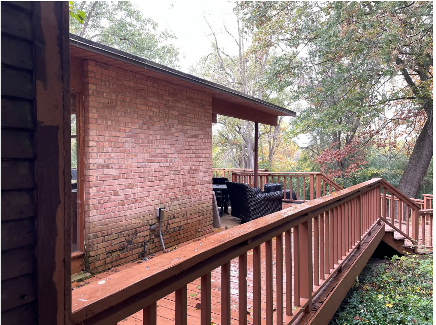
View of proposed project location on the north elevation from the north yard. The shed is visible along the left corner of the picture.
