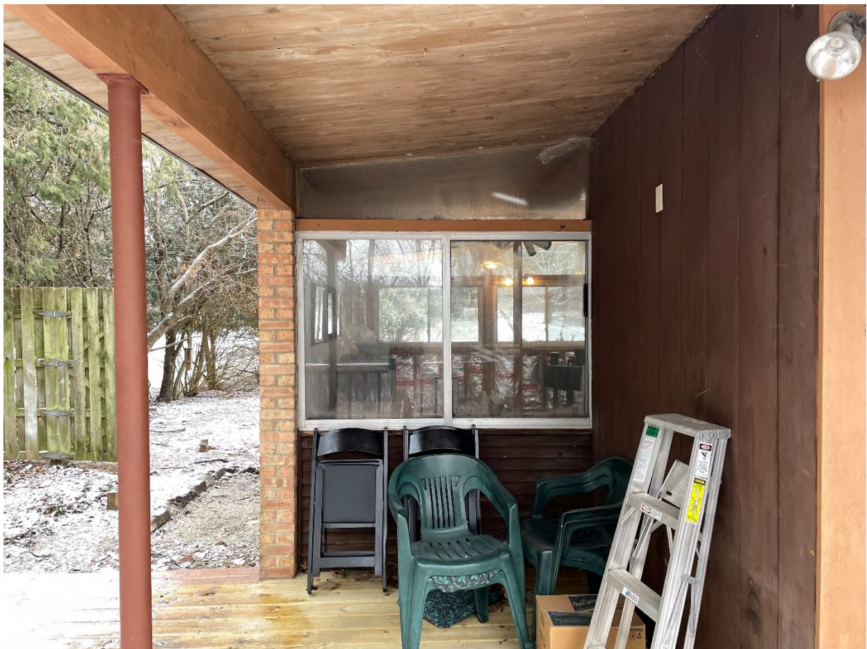
Rear window proposed for replacement; currently original aluminum
