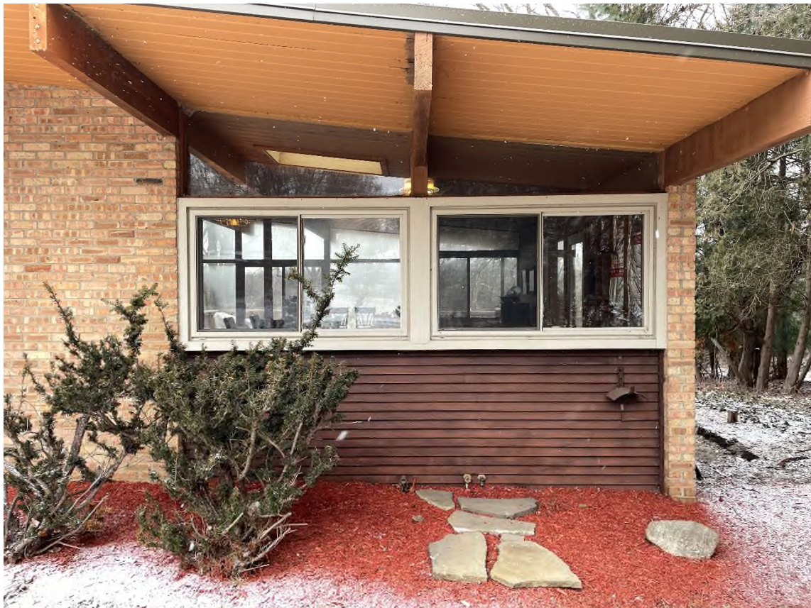
Windows proposed for replacement on front facade; currently vinyl replacement windows
