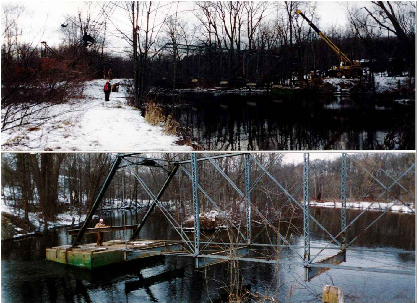
Photos from the Washtenaw County Road Commission show crews using a crane to remove the Bell Road Bridge from its abutments on the Huron River in 1997. Provided by Washtenaw County Road Commission
