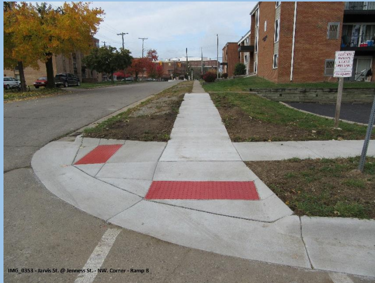
ADA Sidewalk ramps (City of Ypsilanti)
