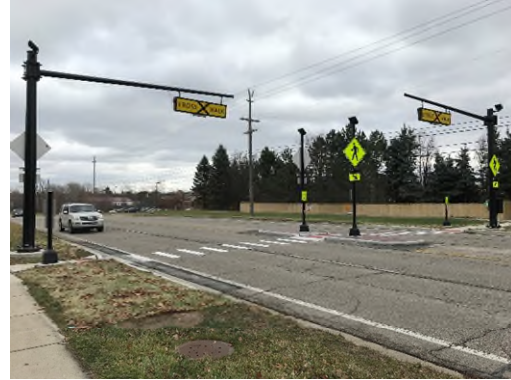
Packard Road Midblock Crossing Installation (Pittsfield Township)
