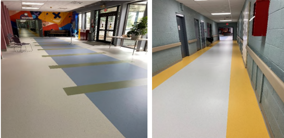
Ypsilanti Township Community Center Flooring Project (2025 E. Clark Road, Ypsilanti Township) 2019 CDBG Priority Project (supplemented by 2017 and 2019 CDBG allocations)
