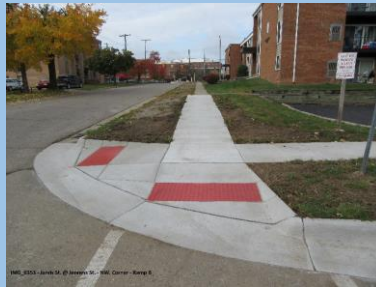
ADA Sidewalk ramps (City of Ypsilanti)
