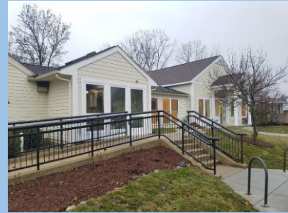
Bryant Community Center Rehab (City of Ann Arbor)
