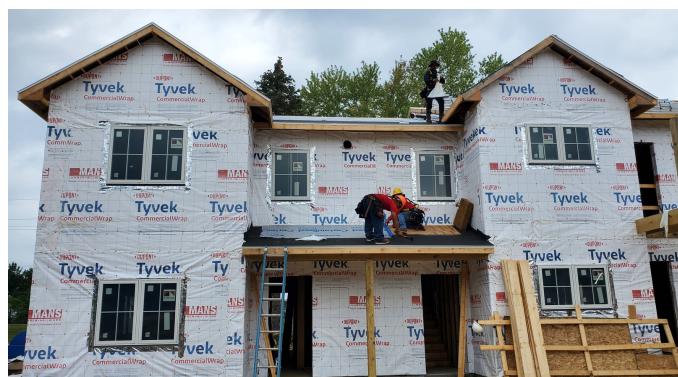
Photo: Hilltop View Apartments construction site
