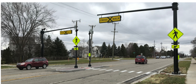
Photo: new mid-block crossing on Packard Road
