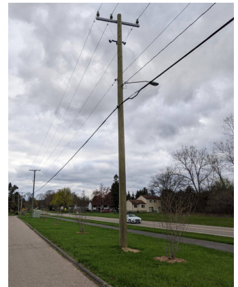
Photo: LED street lights on MacArthur Blvd
