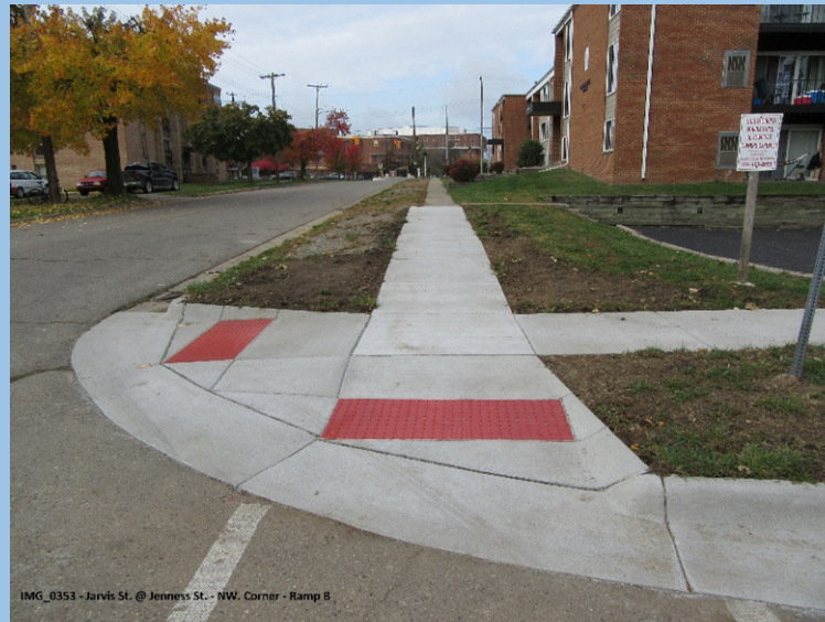
ADA Sidewalk ramps (City of Ypsilanti)
