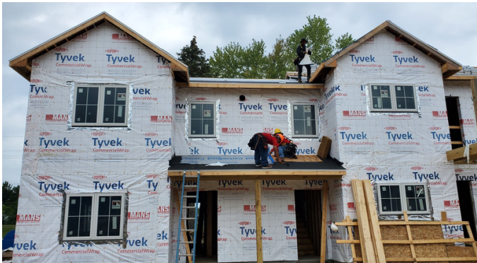
Photo: Hilltop Apartment Construction Site
