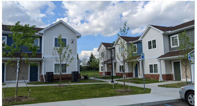
Photo: Completed construction of Hilltop Apartments
