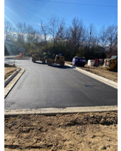
Photo: Construction site of Russell Street Paving & Stormwater Project
