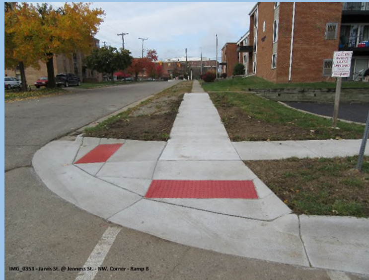
ADA Sidewalk ramps (City of Ypsilanti)
