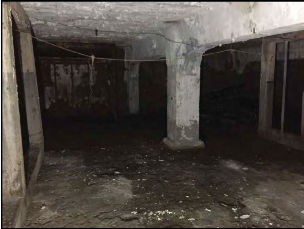
Photo 7: View from basement of the Property building.
