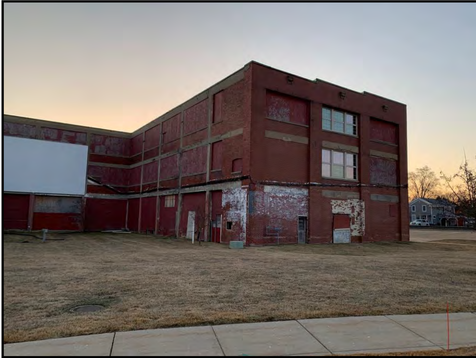
Photo 3: View to the east from the west.
