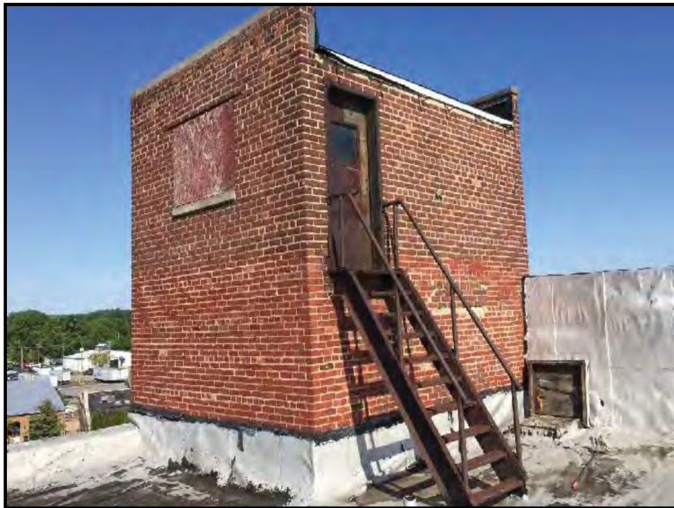
Photo 8: View of the elevator shaft extending from the roof of the Property building.
