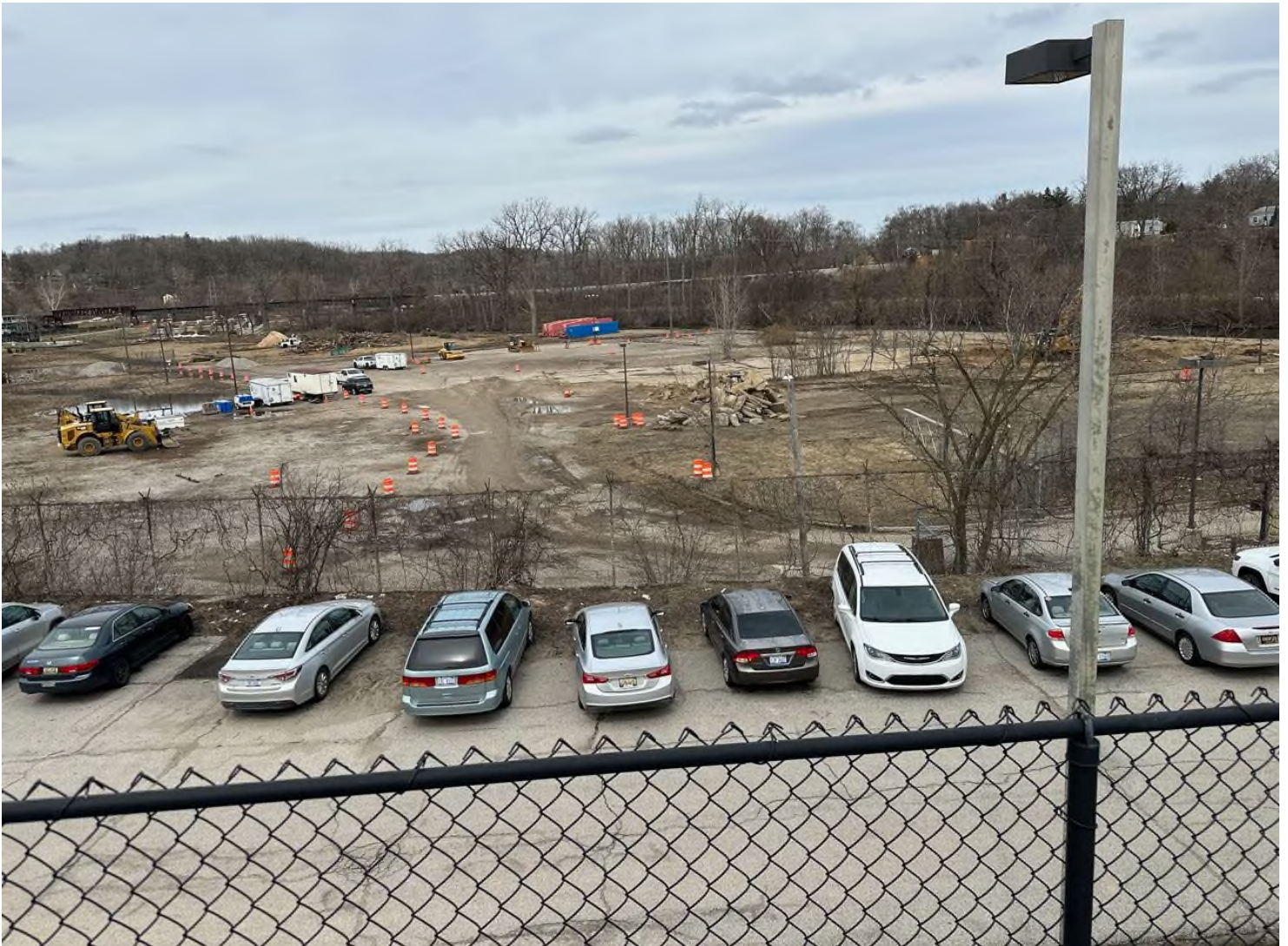
Broadway Park West riverfront redevelopment underway on former DTE Energy site along Huron River north of downtown Ann Arbor on March 28, 2023. Ryan Stanton | The Ann Arbor News
