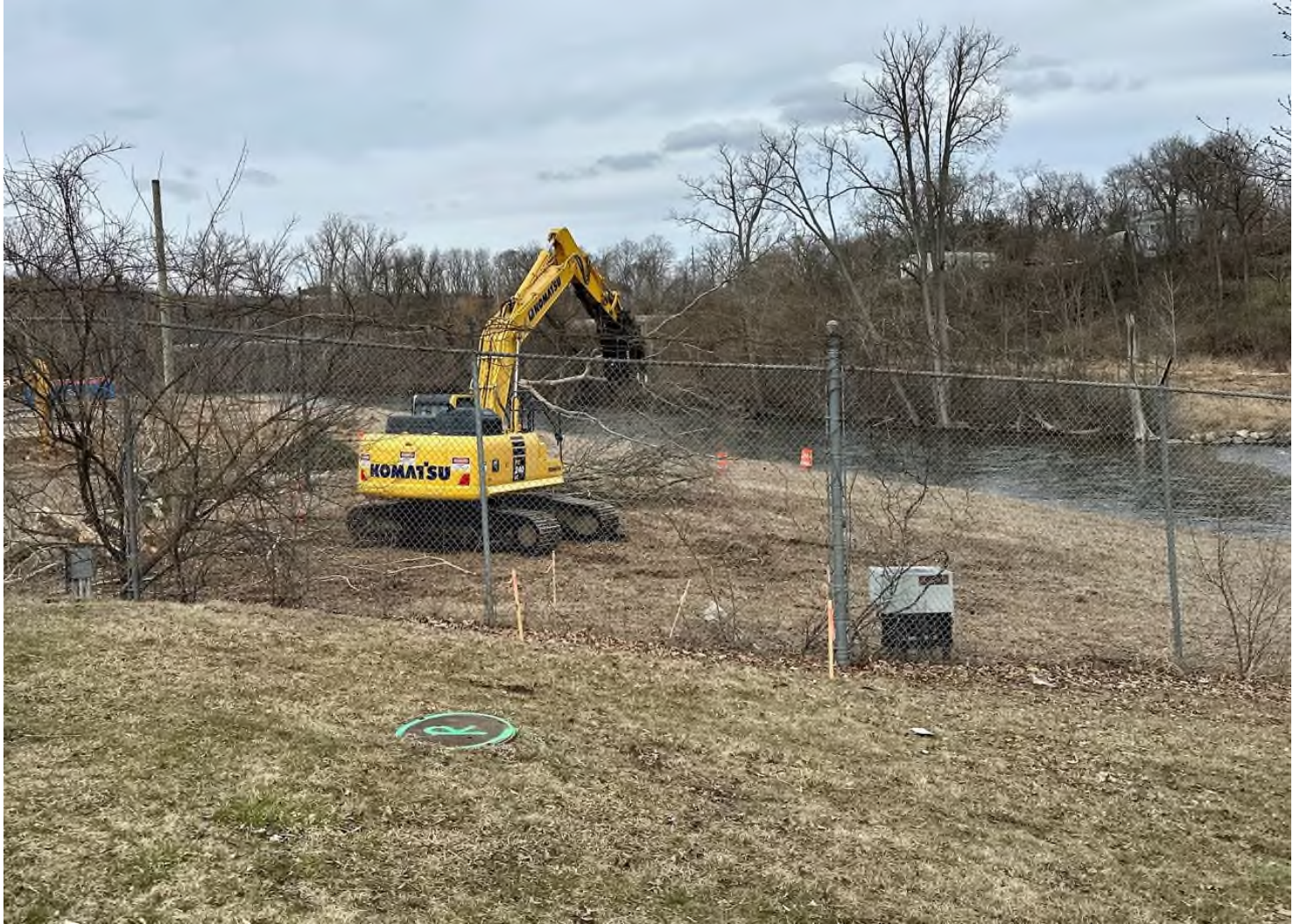
Broadway Park West riverfront redevelopment underway on former DTE Energy site along Huron River north of downtown Ann Arbor on March 28, 2023. Ryan Stanton | The Ann Arbor News
