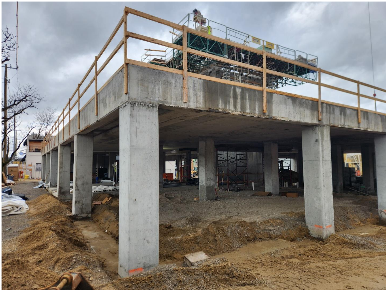
Site Construction Photo from March 5, 2025
