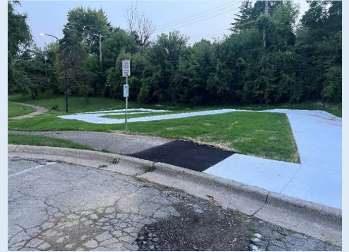
Parkridge Park ADA Pathway Installation (Ypsilanti)
