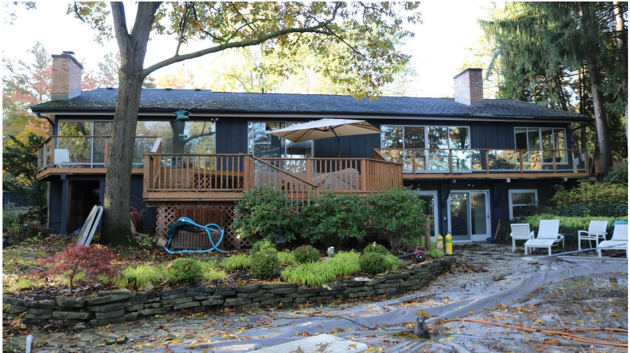
North Elevation (rear of property)
