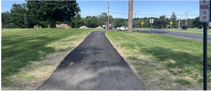
Photo: Construction site of MacArthur Pedestrian Infill Project
