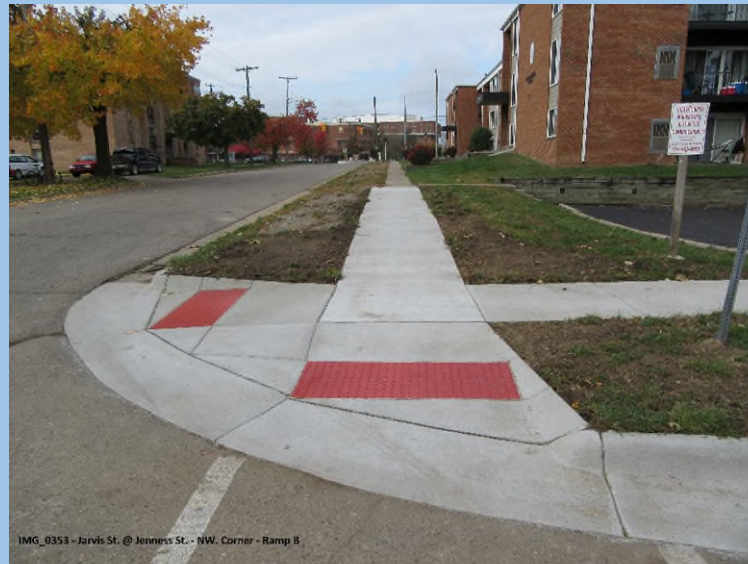
ADA Sidewalk ramps (City of Ypsilanti)
