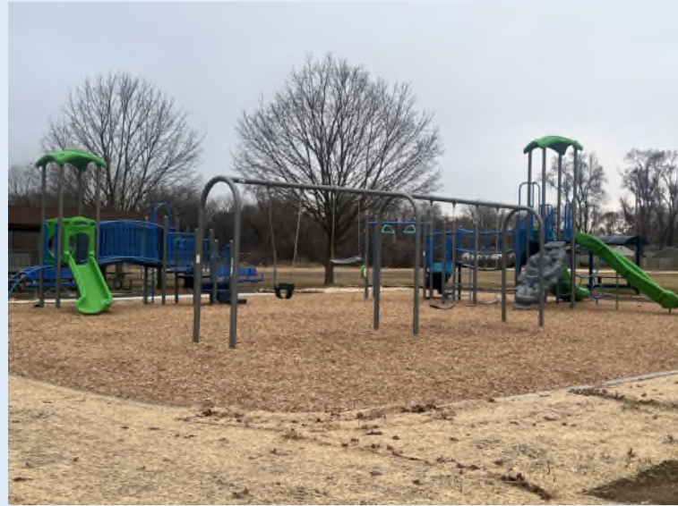
Appleridge Park Playground Renovation (Ypsilanti Township)
